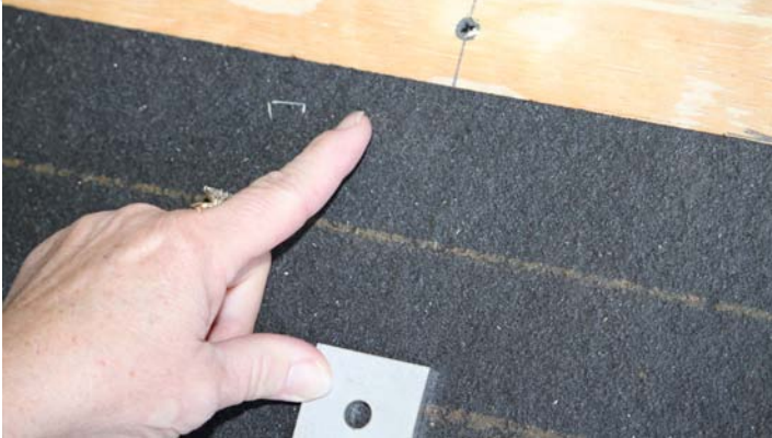
Installation of Asphalt/Bitumen Shingle Roof Hook System: Schletter Part #400847-USA
