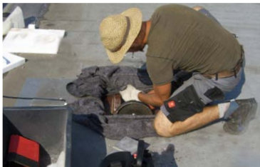
① Opening of the roof cladding
