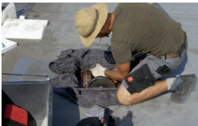
① Opening of the roof cladding
