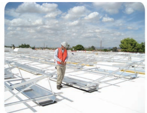
Non-penetrating Windsafe installation
