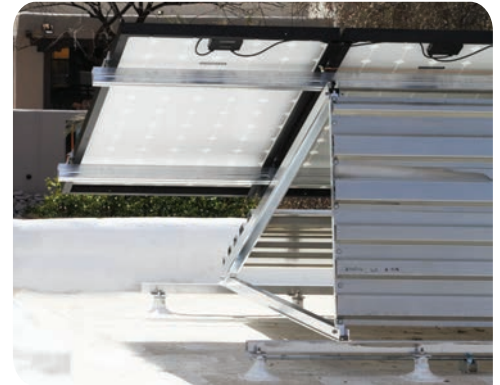
Penetrating Windsafe installation
